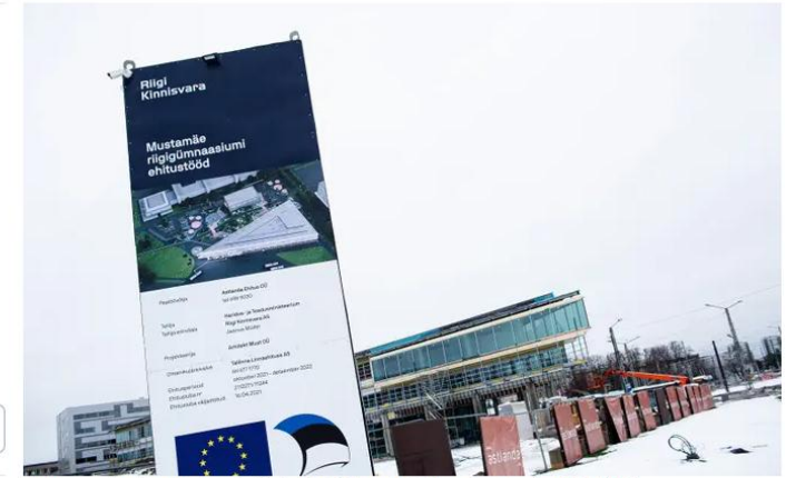
Under-construction Mustamäe State High School in Tallinn. Source: Ken Mürk/ERR
