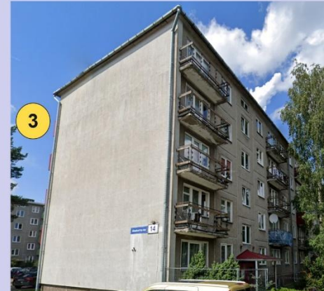
BEMp as the building's exterior walls have been insulated
